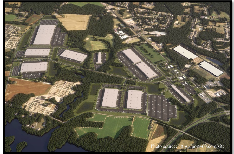
The Port 460 Logistics Center along Pruden Boulevard in Suffolk covers 545 acres and will include about 5 million square feet of warehouse space.
