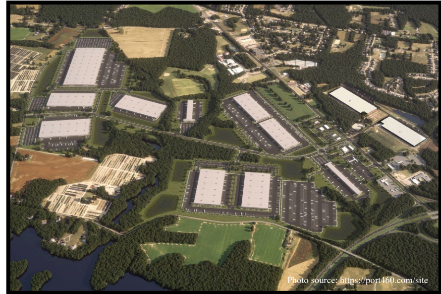
Figure ES-6 – The Port 460 Logistics Center along Pruden Boulevard in Suffolk covers 545 acres and will include about 5 million square feet of warehouse space.
